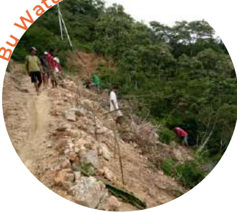
Terrace construction on the slopes of Bu Watuweti
