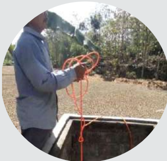
Deepening-of the well in dusun Sidomulyo Desa Sampang
