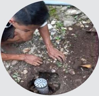
Making of biopore infiltration holes
